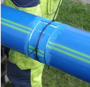
PP- coating ready for welding!
