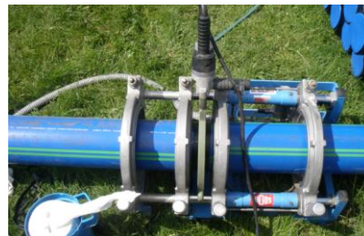
Welding according to standard.
