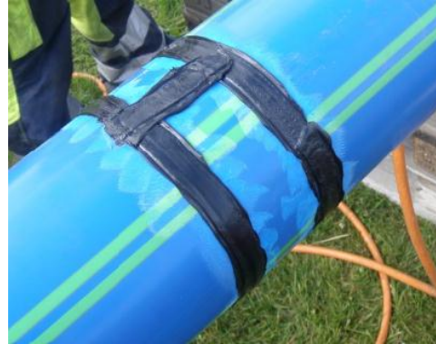
Pipe ready for pipe bursting!
